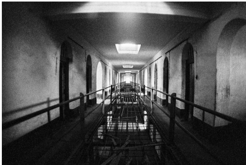
Pudu Prison from the inside.
