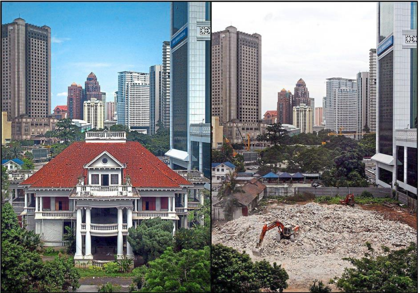
Bok House, before and after photos taken in 2012.
