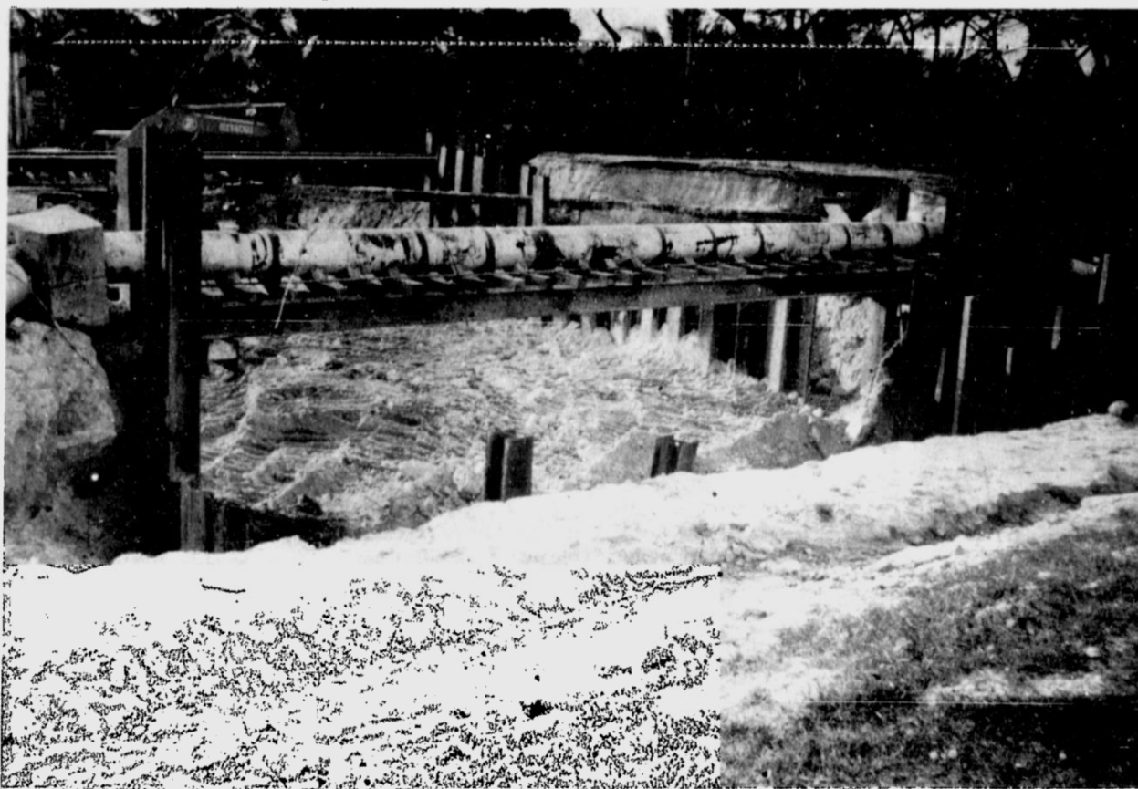
NEW CANAL ... work in progress at Km 3 of the Karak Highway to build a 26-metre twin-box culvert for flood alleviation.
