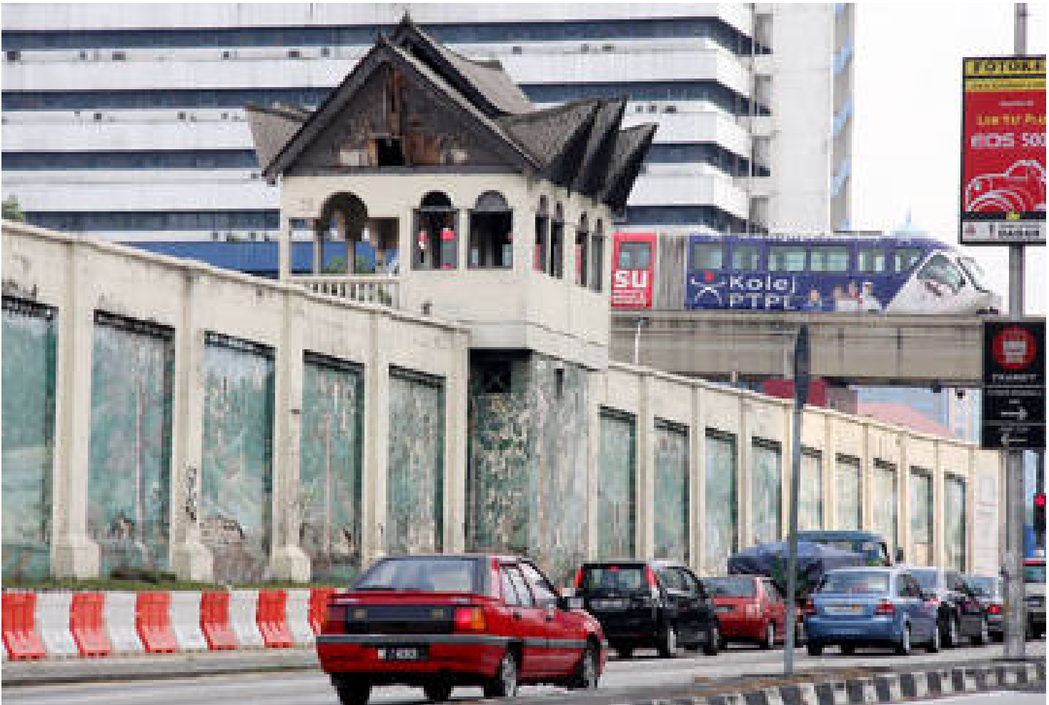
Driving past Pudu Jail side wall on Jalan Pudu will be a distant memory soon for city dwellers after tonight's demolition. - Picture by Choo Choy May
