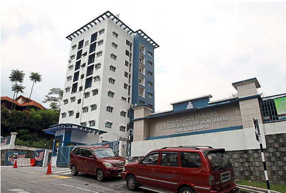
Travers Police Station is the landmark of Jalan Travers.
