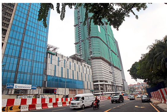
Construction continues along Jalan Travers without any sign of slowing down.
