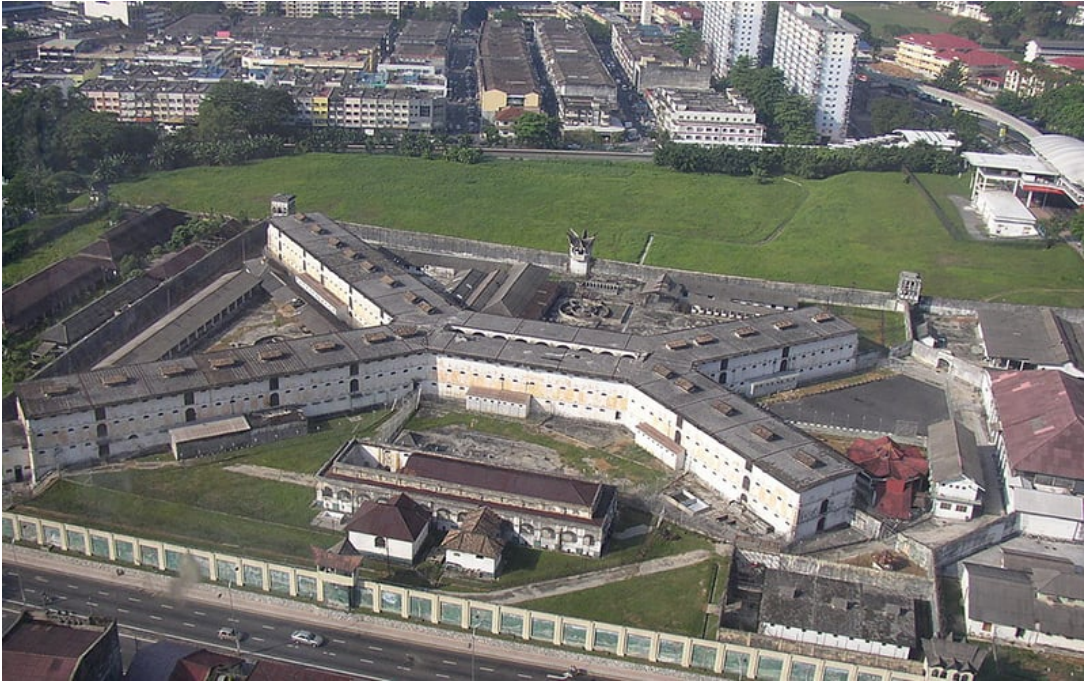
If Pudu Jail had not been demolished, it would have been among the oldest surviving buildings in the country. (Joseph Gan pic)
